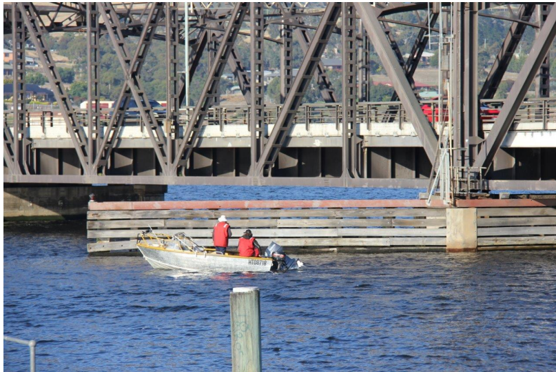
Figure 4. Bridgewater Bridge closed lift span. Photo supplied by New Bridgewater Bridge Project.
