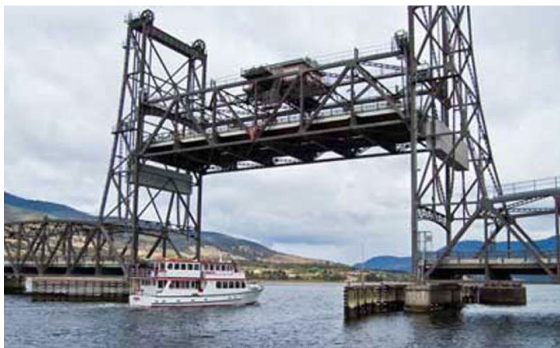
Figure 5. Bridgewater Bridge open lift span. Photo: Ian D Cooper.
