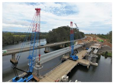
This is an example of what a temporary bridge can look like. Temporary bridges enable the movement of material and equipment to support the construction of new bridges.
