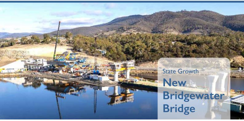
Concrete bridge segment placement on the Granton side of the River Derwent is ramping up with the recent commissioning of the project's second set of Special Segment Lifting Devices.
