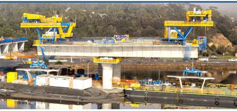
Segment erection is progressing from both foreshores toward the middle of the River Derwent. This image shows the Special Segment Lifting Devices (SSLDs) on the Granton side lifting segments from the deck of the temporary bridge.
