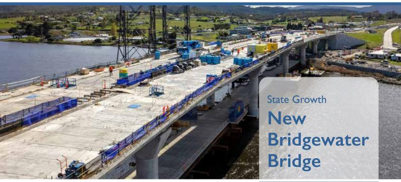
Significant progress has been made on the erection of concrete bridge segments that will form the new bridge deck. Finishing works continue with the installation of the new bridge barriers.
