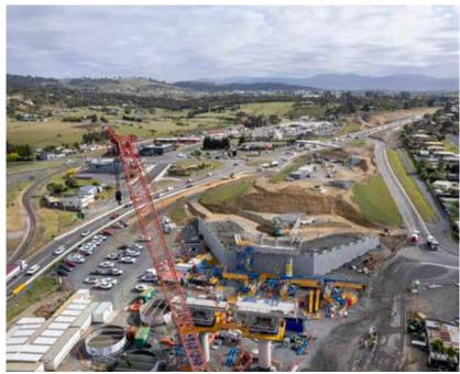
Above: Construction of the northern approach to the new bridge is progressing. The northern abutment stands in front of the reinforced soil slope (RSS) walls, showing the new alignment of the Midland Highway. The grassed batters of the bridge's northern approach prevent erosion and minimise any dust impact on the local community.
