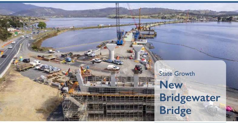
The new bridge sub structure is progressing well on the Granton side of the River Derwent, including the recent concrete pouring of the southern abutment, ongoing piling and construction of the piers. All of the land piers on the northern and southern sides of the river have now been completed.
